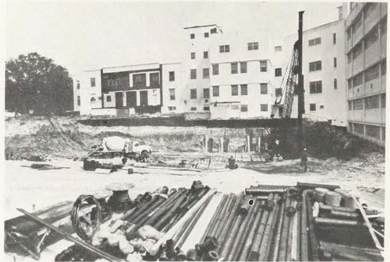
The old Maternity porches gave way to progress (left) when Misener Marine sub-contracted to drive the 784 pilings needed to support the Witt Memorial Building.
