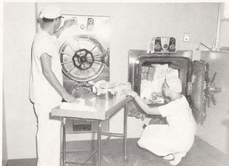
Autoclaves "Elmer" (left) and "Elsie" (right), installed in the new surgery opened during May 1951, were used as sterilizers by all the hospital departments.
